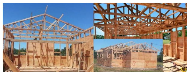
Figura 8. Colocación de tímpanos, cabriadas y tableros fenólicos faltantes. Figure 8. Positioning of trusses and phenolic boards.
