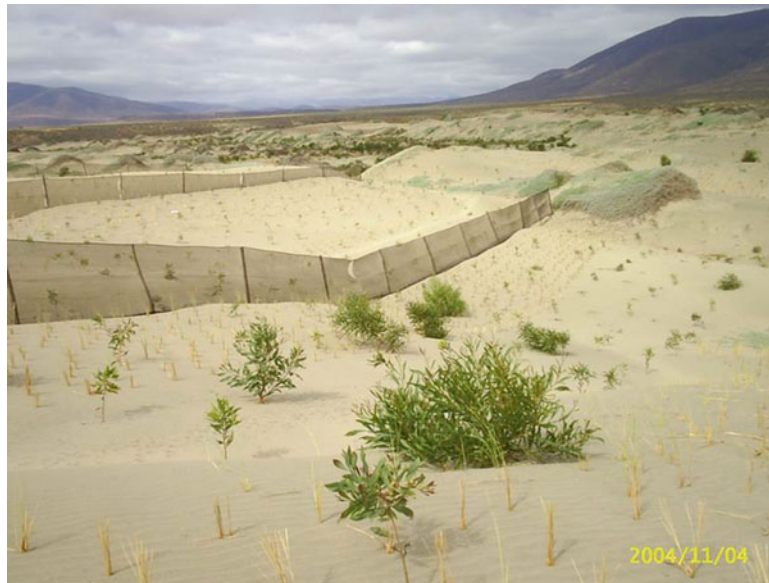
Fig. 7.1 Dunes control work in Huentelauquén farm. Province of Choapa, Coquimbo Region. Lat 31°37'38" S and Long 71°33'03" W (Source: Patricio Rojas 2004)
